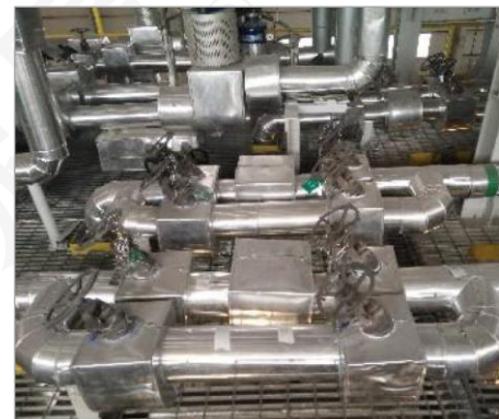
减温减压蒸汽管道气凝胶保温
