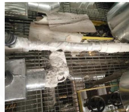
减温减压蒸汽管道气凝胶保温
